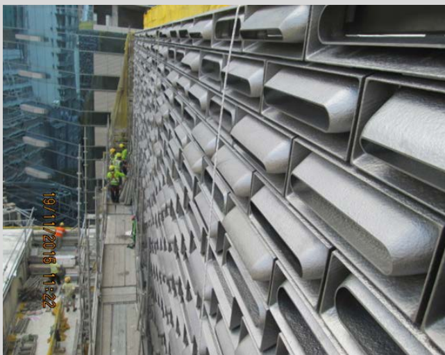
Arbuthnot Auditorium - North Facade
