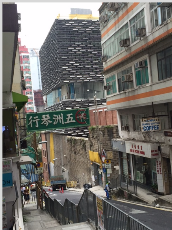
SW Corner View - Old Bailey Street
