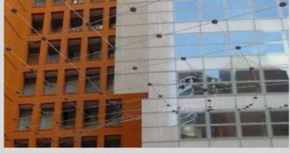
Aurora Place features cast football and hamburger shaped nodes which transfer high tension loads in a laced single catenary structure. Prodigious tension detailing delivers a world-first overhead CBD piazza canopy.
